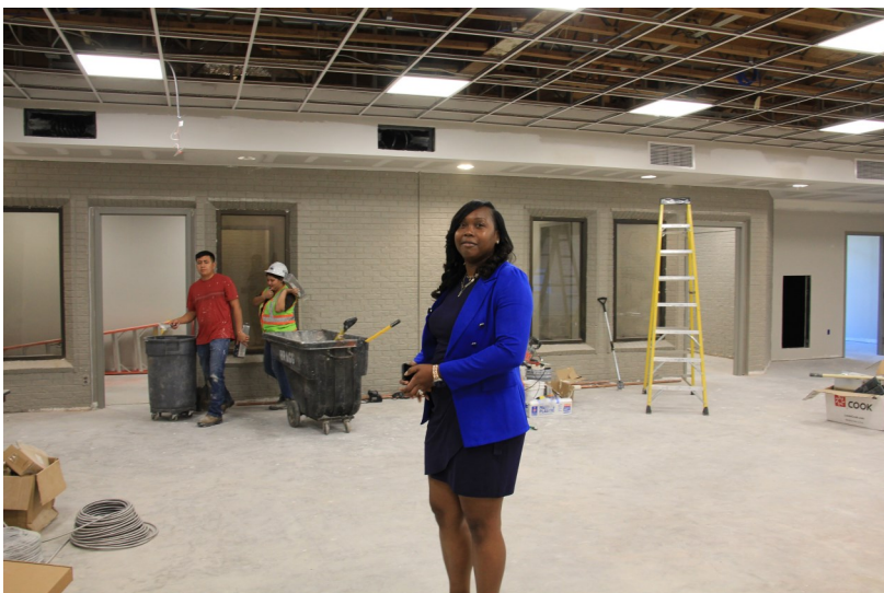
CCID Court Clerk Dr. Bryana Smith McDougal surveys work that will convert a former bus station lobby into a courtroom.
